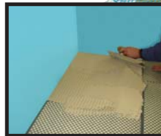
6. Cover Plastic Ply with Nicobond Rapidflex adhesive
