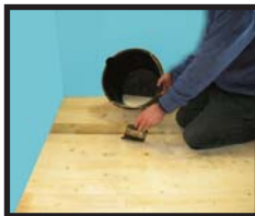
2. Prime timber and allow to dry
